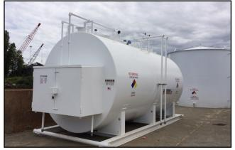
12,000 Gallon Single-Wall Dual Compartment Tank on skids
