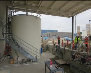
$12^{\circ}$  x 15 ft. tall Vertical UL tank with spiral staircase and top handrail
