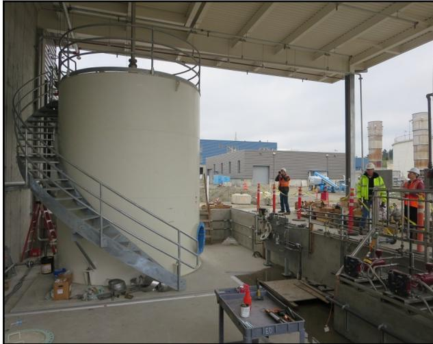
12' x 15 ft. tall Vertical UL tank with spiral staircase and top handrail
